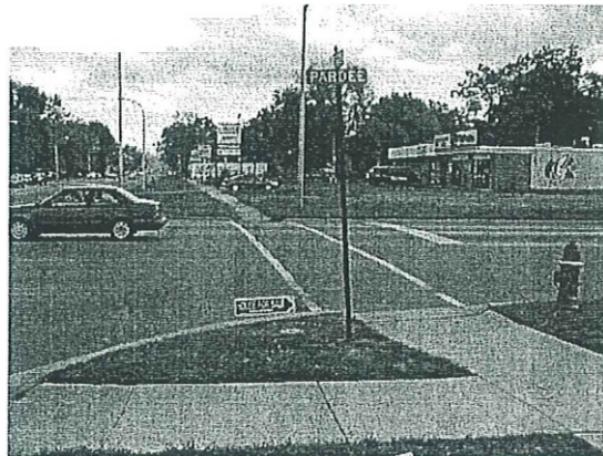
Improvements to the public infrastructure, including sidewalks and crosswalks within the public right-of-way, are necessary to encourage orderly growth and economic expansion within the DDA Development District.
