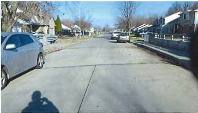
Document Name: RIMG3005.JPG Category: Approach Span Number: Comments: South approach looking north
