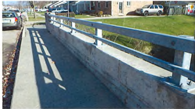
Document Name: RIMG3011.JPG Category: Railing Span Number: Comments: West railing
