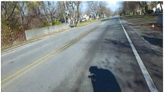
Document Name: RIMG3049.JPG Category: Approach Span Number: Comments: South approach looking north
