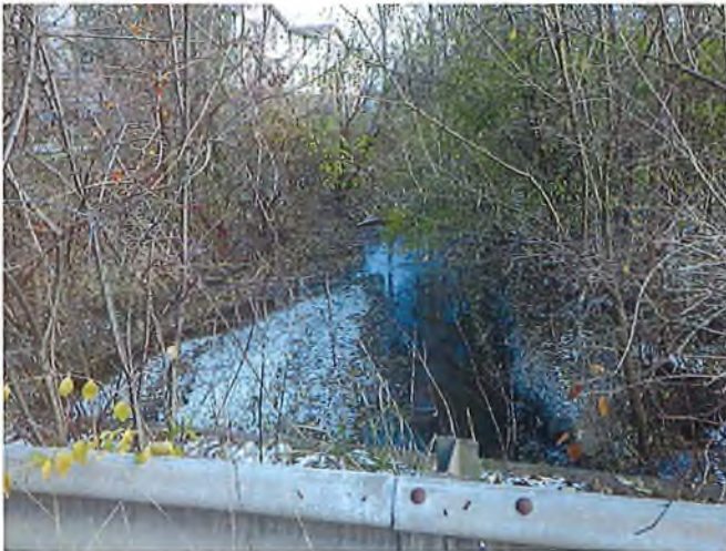
Document Name: RIMG2873.JPG Category: Channel Span Number: Comments: Channel looking west
