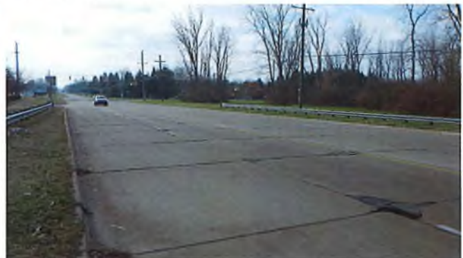
Document Name: RIMG2967.JPG Category: Approach Span Number: Comments: south approach looking south
