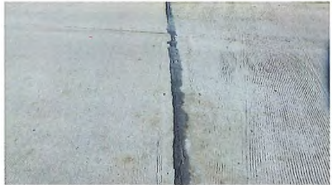
Document Name: RIMG3020.JPG Category: Joints Span Number: Comments: East joint
