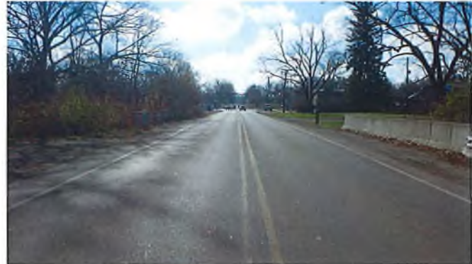
Document Name: RIMG3058.JPG Category: Approach Span Number: Comments: north approach looking south
