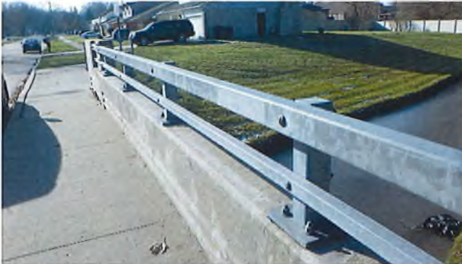
Document Name: RIMG3023.JPG Category: Railing Span Number: Comments: East railing
