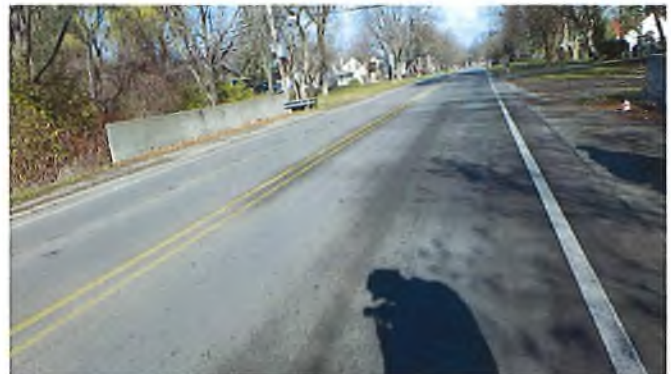
Document Name: RIMG3049.JPG Category: Approach Span Number: Comments: South approach looking north
