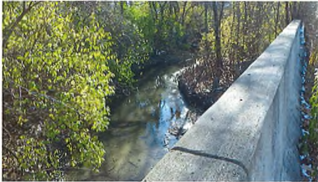
Document Name: RIMG3057.JPG Category: Channel Span Number: Comments: Channel looking west
