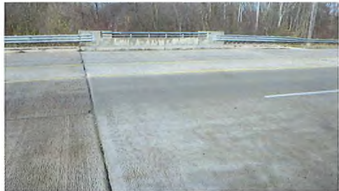
Document Name: RIMG2971.JPG Category: Joints Span Number: Comments: West joint
