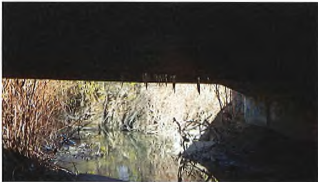
Document Name: RIMG3076.JPG Category: Span Number: Comments:
