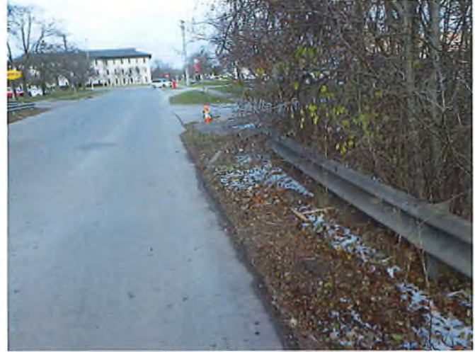
Document Name: RIMG2874.JPG Category: Railing Span Number: Comments: East guardrail
