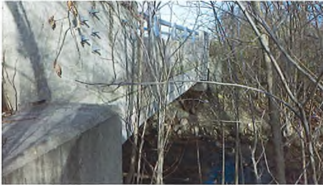
Document Name: RIMG2986.JPG Category: Elevation Span Number: Comments: West fascia
