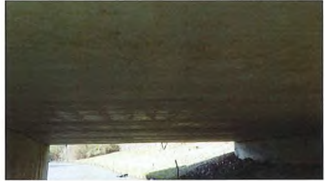
Document Name: RIMG3035.JPG Category: Superstructure Span Number: Comments: Box beams/deck bottom
