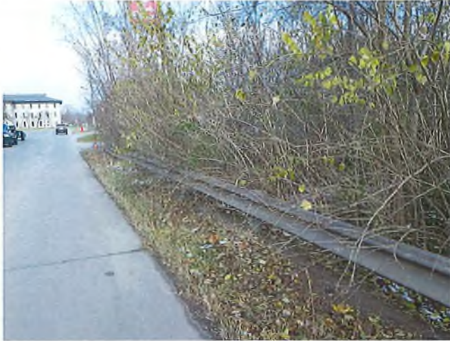
Document Name: RIMG2871.JPG Category: Railing Span Number: Comments: West guardrail
