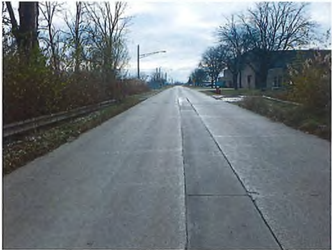
Document Name: RIMG2870.JPG Category: Approach Span Number: Comments: South Approach looking south
