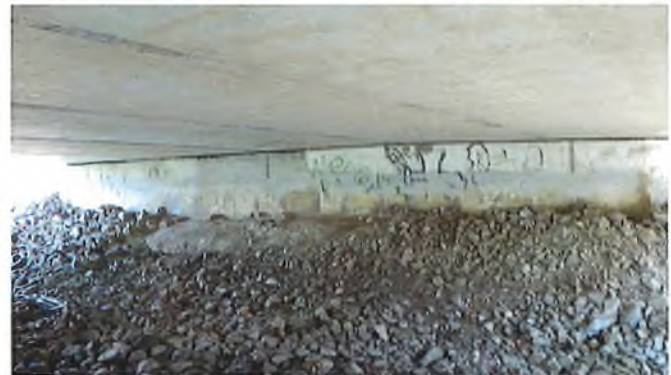
Document Name: RIMG3037.JPG Category: Substructure Span Number: Comments: North abutment
