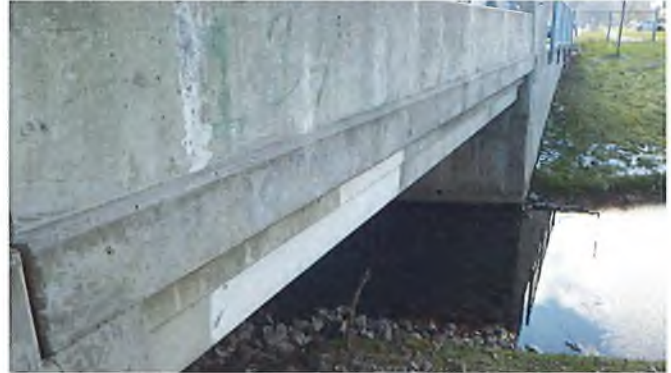
Document Name: RIMG3041.JPG Category: Elevation Span Number: Comments: west fascia
