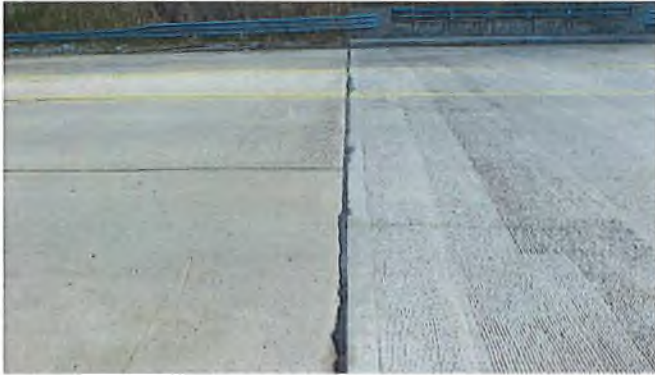
Document Name: RIMG2980.JPG Category: Joints Span Number: Comments: East joint
