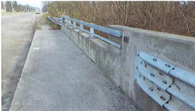
Document Name: RIMG2970.JPG Category: Railing Span Number: Comments: West railing
