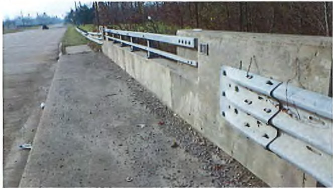
Document Name: RIMG2979.JPG Category: Railing Span Number: Comments: East railing
