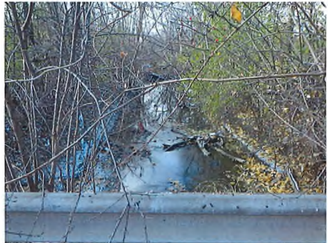
Document Name: RIMG2879.JPG Category: Channel Span Number: Comments: Channel looking east
