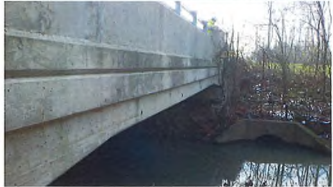
Document Name: RIMG2999.JPG Category: Elevation Span Number: Comments: East Fascia
