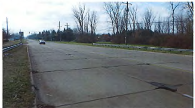
Document Name: RIMG2967.JPG Category: Approach Span Number: Comments: south approach looking south
