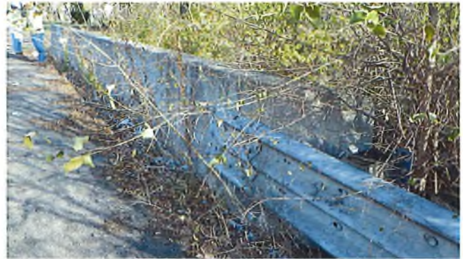
Document Name: RIMG3052.JPG Category: Railing Span Number: Comments: West railing
