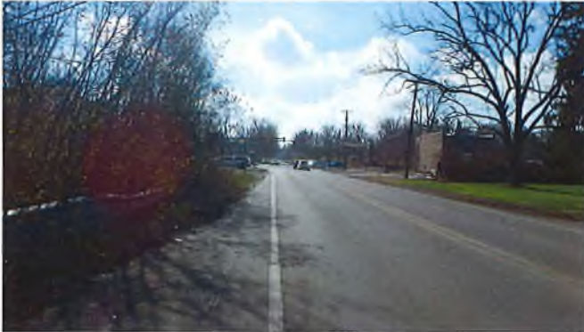
Document Name: RIMG3050.JPG Category: Approach Span Number: Comments: south approach looking south
