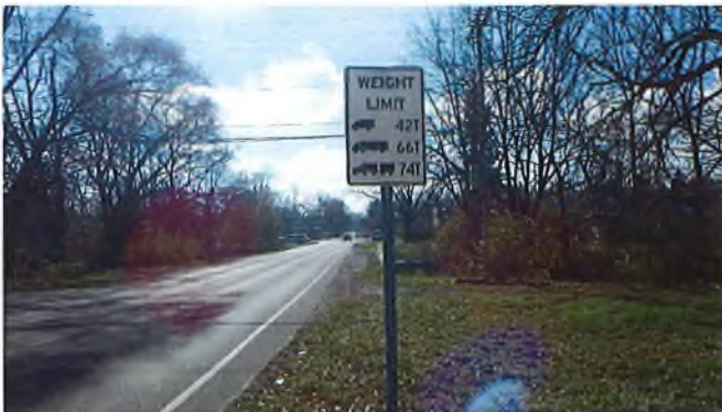
Document Name: RIMG3060.JPG Category: Posting Span Number: Comments: 42T/66T/74T load posting sign at north approach
