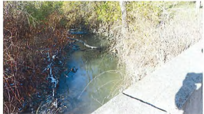
Document Name: RIMG3065.JPG Category: Channel Span Number: Comments: channel looking east
