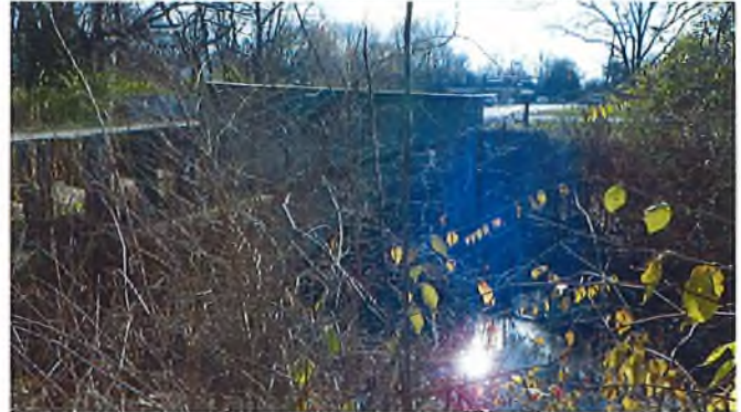
Document Name: RIMG3080.JPG Category: Elevation Span Number: Comments: west fascia
