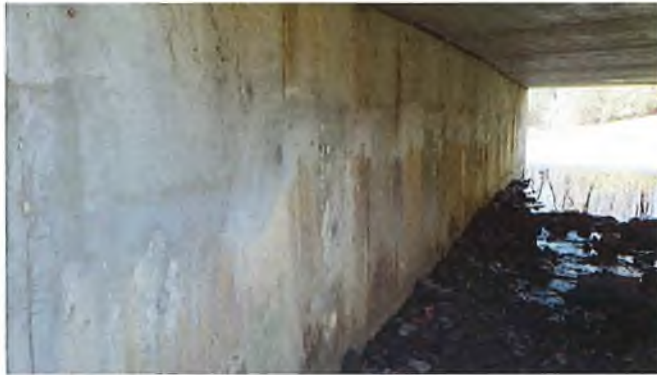
Document Name: RIMG3033.JPG Category: Substructure Span Number: Comments: South abutment
