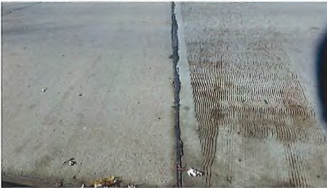
Document Name: RIMG3010.JPG Category: Joints Span Number: Comments: West joint
