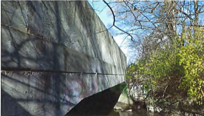
Document Name: RIMG3068.JPG Category: Elevation Span Number: Comments: east fascia
