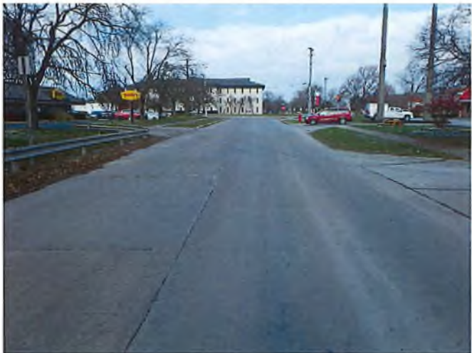
Document Name: RIMG2876.JPG Category: Approach Span Number: Comments: North approach looking north
