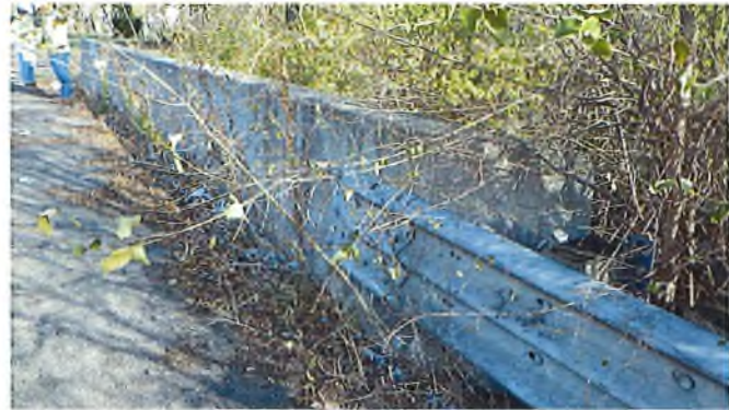
Document Name: RIMG3052.JPG Category: Railing Span Number: Comments: West railing
