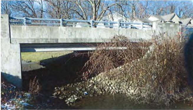
Document Name: RIMG3031.JPG Category: Elevation Span Number: Comments: east fascia
