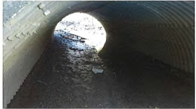
Document Name: RIMG2888.JPG Category: Culvert Span Number: Comments: south barrel
