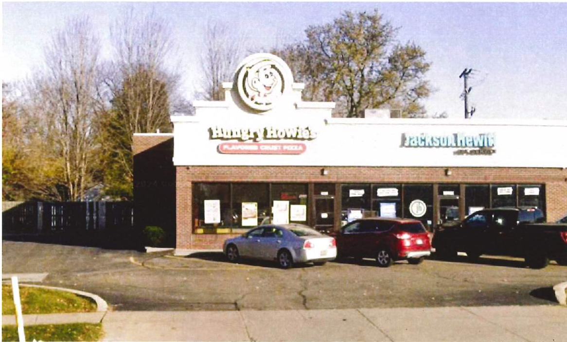
EXISTING FRONT FACADE
